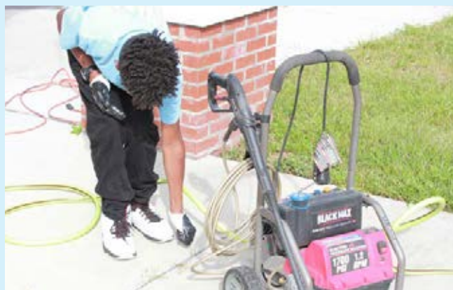
Removing the weeds in the crack before pressure washing
